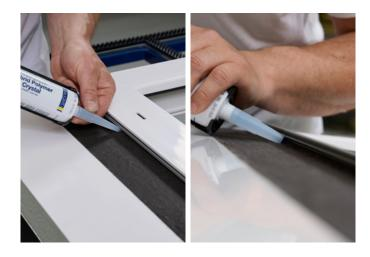
**Important:** With floor thresholds, make sure that the water drip edge remains open: only seal the front threshold cavity with blaugelb Hybrid Polymer Crystal 40 mm from the outer edge of the corners. Remove any protruding material.
