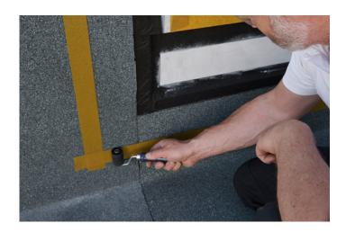
The figure shows the completed masking on an example window frame with plinth thermal insulation profile, installation in the supporting wall structure (monolithic installation).
