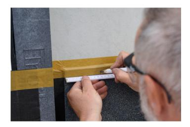
Now mask off the marked area using blaugelb FLK Masking Tape (25 or 50 mm), ensuring a clean and straight application. Press on the blaugelb FLK Masking Tape with the blaugelb Pressure Roller (item no. 9074068) to prevent water ingress from behind.
