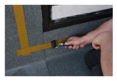
Step 4: Additionally mask off the window frame in the area of the window frame (width 30 mm, height 150 mm from outer covering UE) with a second layer of masking tape (blaugelb FLK Masking Tape 25 mm).
