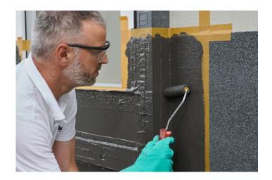
Tip: Stand up for a second and view the sealed surface from a slight distance. Changing your perspective quickly identifies any defects.
