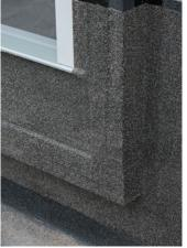
We recommend covering the sealed surface with an additional protective layer (e.g. plastic non-woven 300  $g/m^2$ ) to protect it against mechanical abrasion (e.g. by stones) when the soil is deposited onto the plinth.
