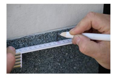
The 100 mm overlap starts from the existing building waterproofing and is marked with a pencil.
