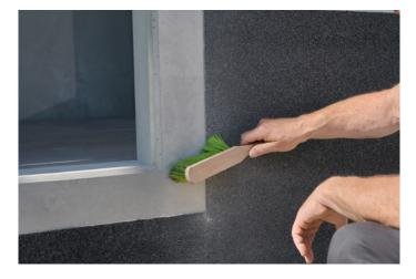
All protective foils on the substrates must be removed in the area of the sealing.
