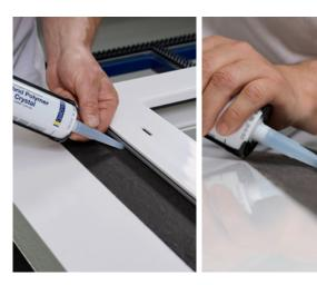
**Important:** With floor thresholds, make sure that the water drip edge remains open: only seal the front threshold cavity with blaugelb Hybrid Polymer Crystal 40 mm from the outer edge of the corners. Remove any protruding material.
